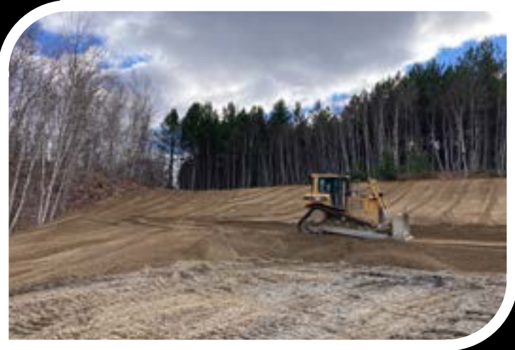
Slopes stabilization (October 2022)
