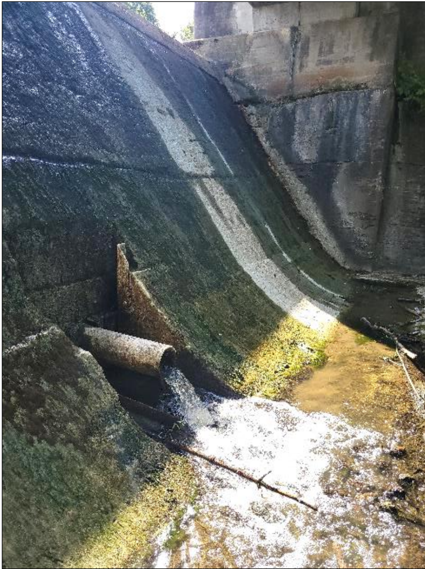
Low flow pipe in spillway
