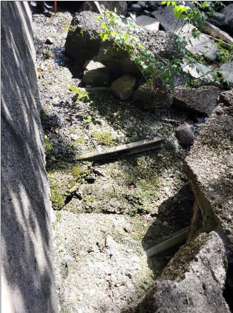
North wingwall apron/footing with lateral lengths of steel rails visible
