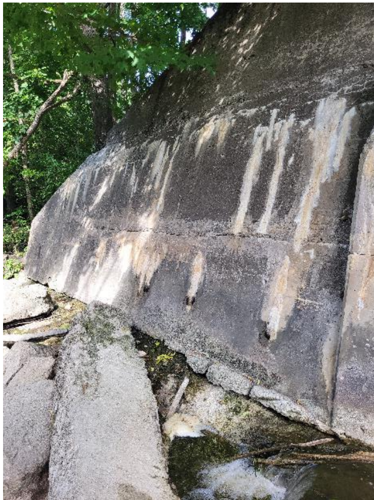
North wingwall concrete missing from interface between wingwall bottom and top of apron
