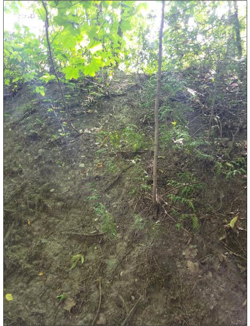
Downstream embankment with bare ground
