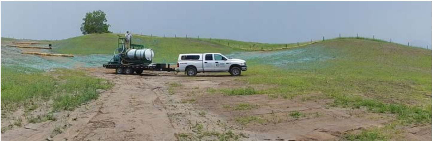
Figure 1: A truck towing a slurry of seed, ProGanics, Fertilizer and Tackifier (erosion control product) and a worker hydraulically applying over the finished grade of a legacy site.
